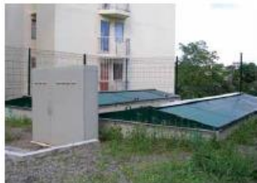
Plateau Tiberge (Martinique), 400 PE. Ecodisk installed right next to homes
